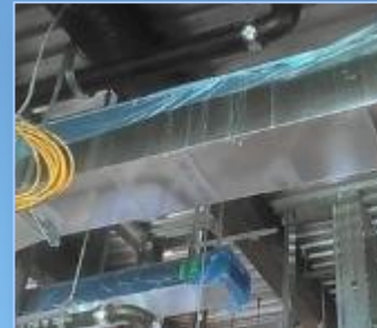
Ductwork Protected from water/debris
