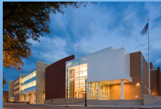
Broughal Middle School
